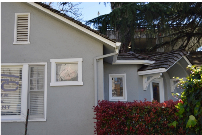
Figure 3. View of smaller typical smaller fixed wood windows at west elevation.
