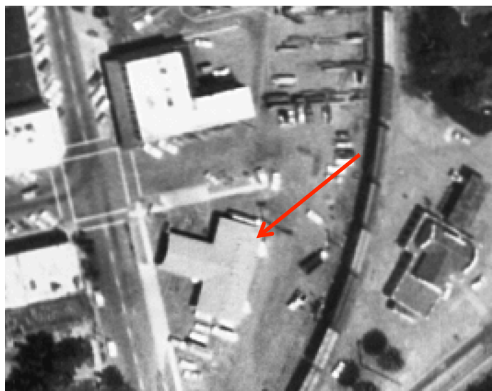
Figure 6. 1965 aerial photograph showing T-plan subject building without additions of more recent origin. (UC Santa Barbara Library, Frame Finder, Cartwright Aerial Surveys, CAS-65, 130, Frame 14-213)
