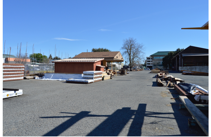
Figure 2. View of asphalt paved lumberyard and ancillary shed buildings within the lumberyard.
