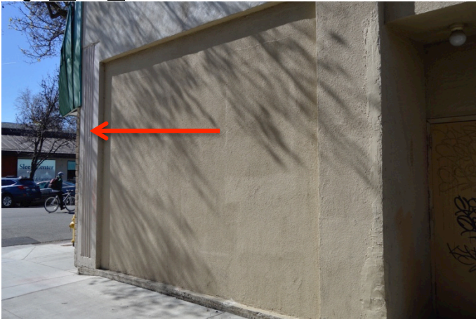
Figure 1. East, alley facing elevation. Red arrow points to formed concrete Art Deco detail at corner. Looking south.
