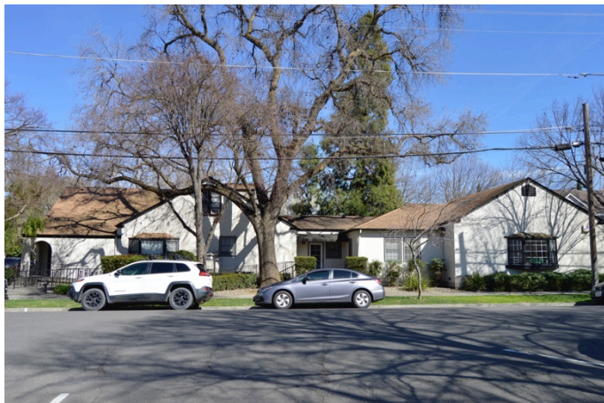
Figure 1. 500 4th Street viewed from D Street, looking east. Building historically addressed 502 4th Street (left) and 1988 hyphen and addition (right)
