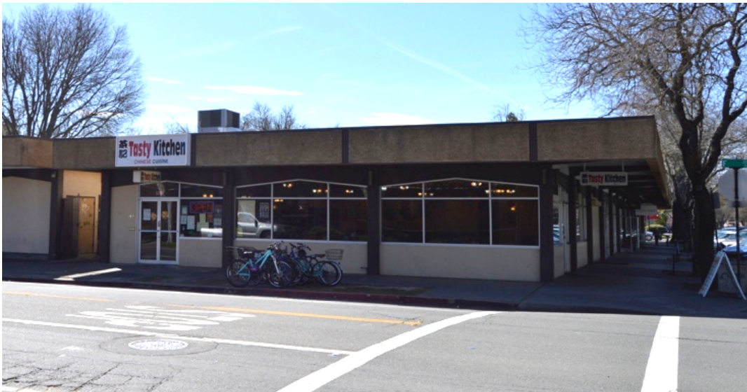
Figure 2. Storefronts facing F Street and 4th Street within portion of building addressed 612 4th Street, looking west.
