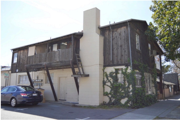
Figure 1. East elevation viewed from 4th Street, looking southwest.
