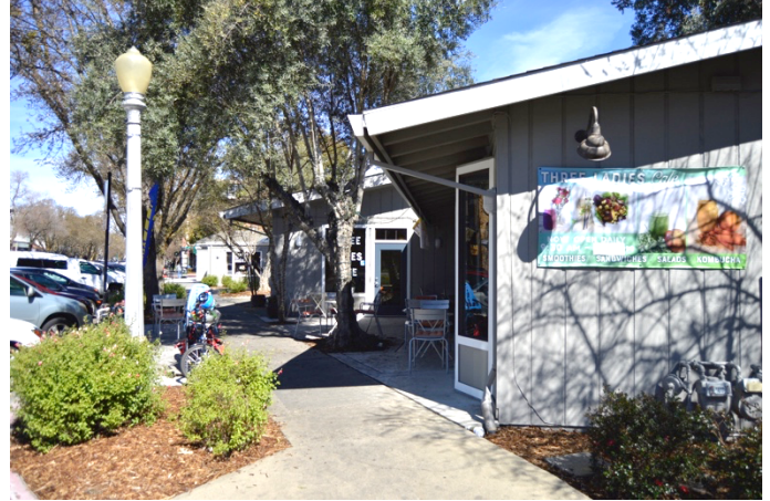
Figure 2. Overhanging roof eaves viewed from east side of F Street, looking north.
