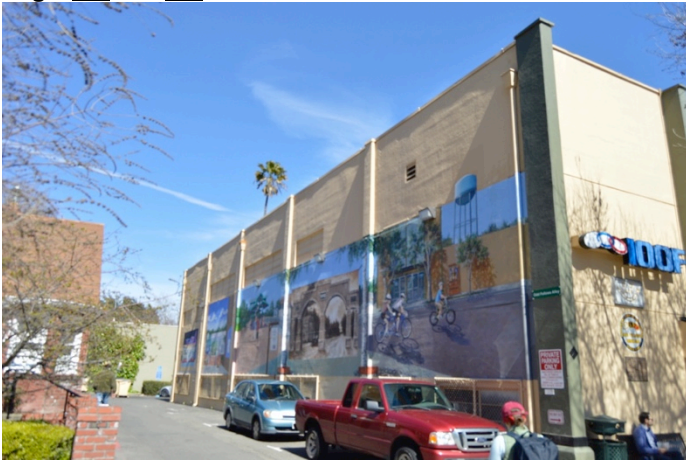
Figure 1. West elevation of 415 2nd Street viewed from 2nd street, looking north.
