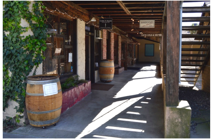
Figure 2. Passageway to storefronts at first story of west elevation, looking south.
