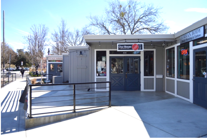
Figure 1. Typical one-story storefront with contemporary paneled doors and rectangular sidelites, visible at the north and west elevations.
