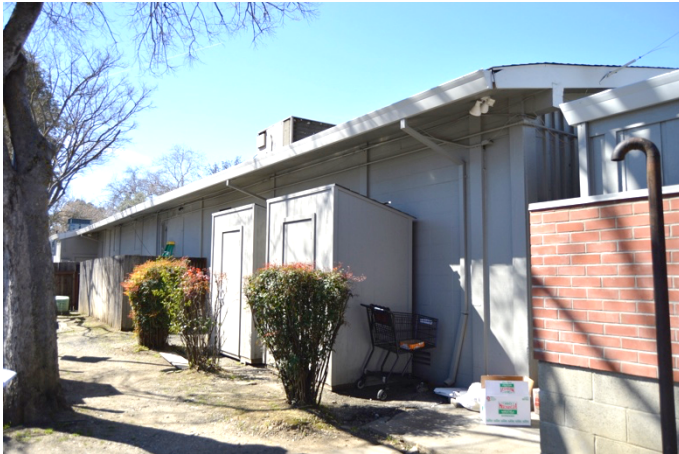
Figure 3. Rear of building is not fenestrated.
