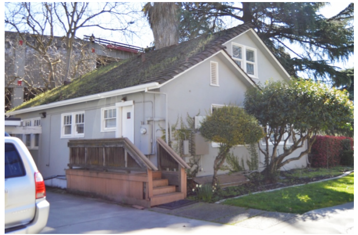
Figure 2. North elevation adjacent to driveway, looking southeast.
