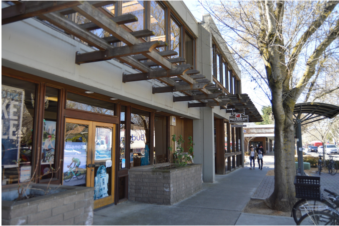
Figure 1. East storefront and adjacent planters, looking west.
