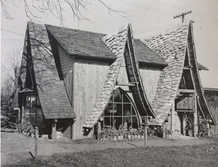
Figure 2. Subject building photographed in 1949 (Lofland and Haig, Images of America: Davis 1910s-1940s , image credited to Mickey Barlow)
