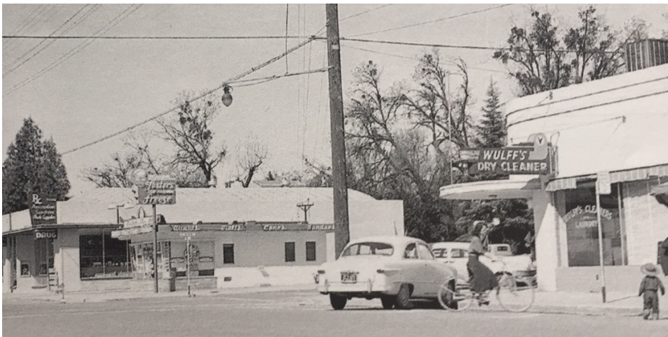
Figure 3. 703-705 2nd Street pictured at right, 1951. The south elevation of the subject building was altered by 1951 with a corner entrance and curved canopy, emphasizing the streamlined facade of the building. ((Lofland and Haig, Images of America: Davis 1910s-1940s . Amended by author)
