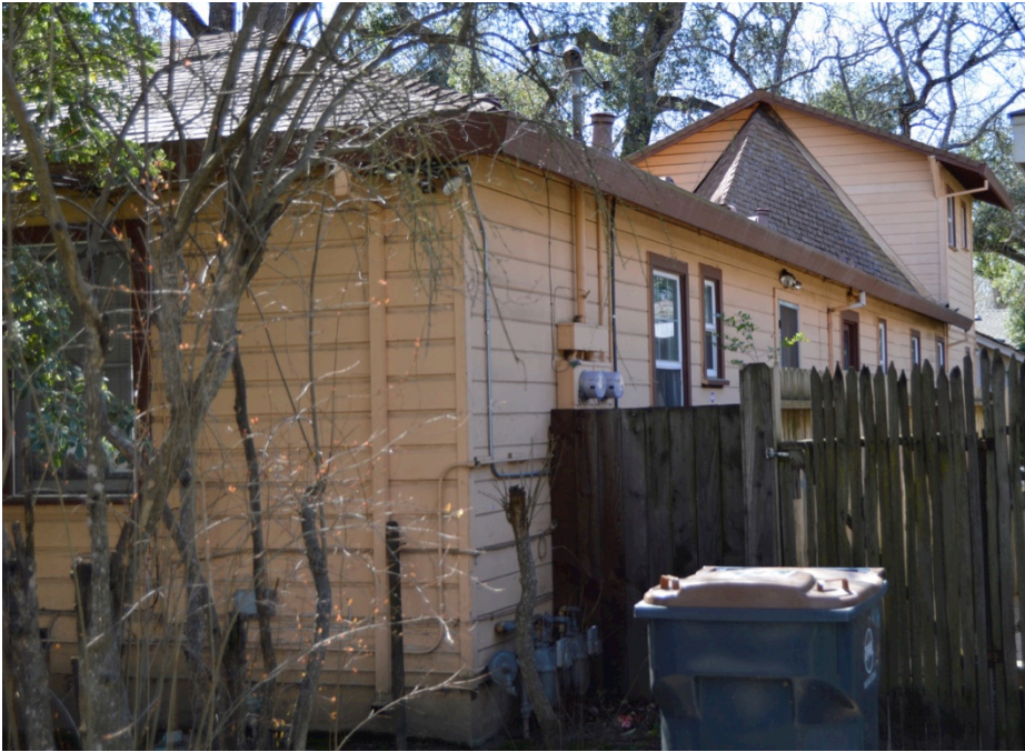
Figure 1. North elevation and rear, two-story addition, looking west.
