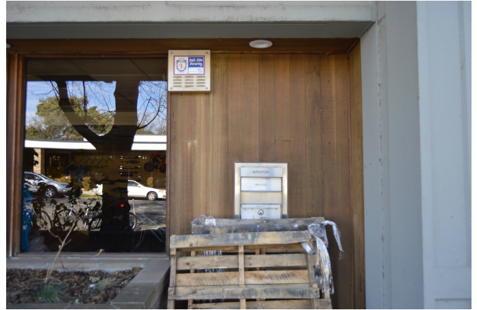
Figure 2. Deposit box at west end of east storefront, looking south.
